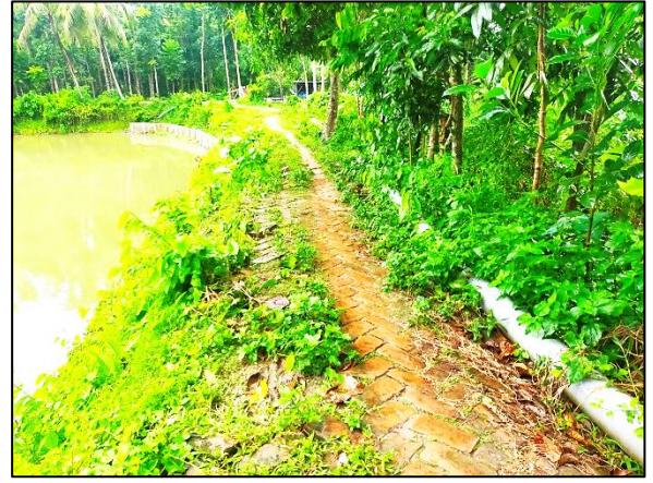
Road-206, Naria Pourashava
