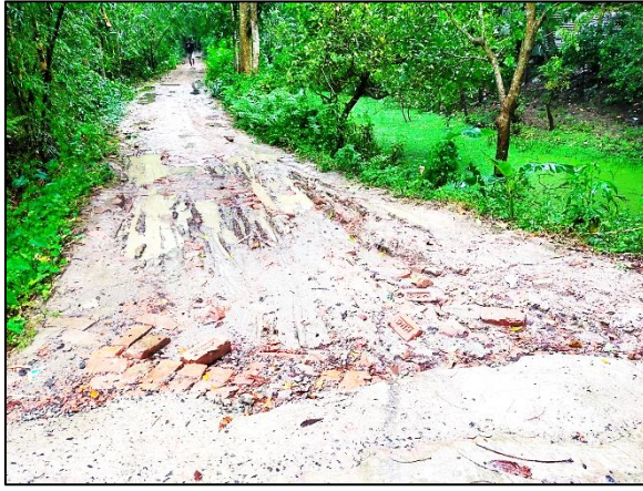
Road-206, Naria Pourashava
